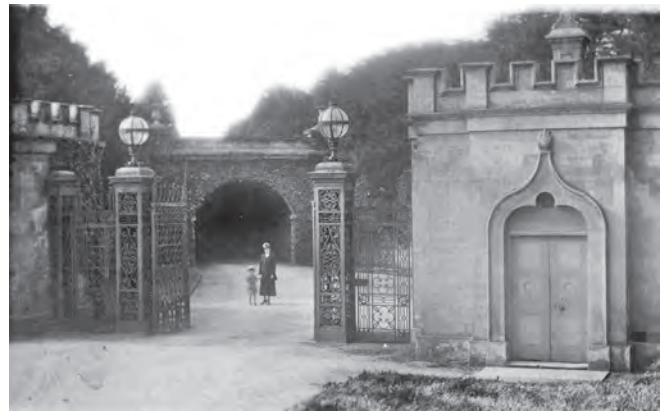
The tunnel entrance near the new service block
